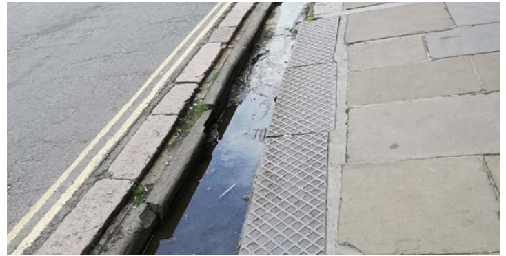
Image 24: Lack of Quality & Consistent Materials
