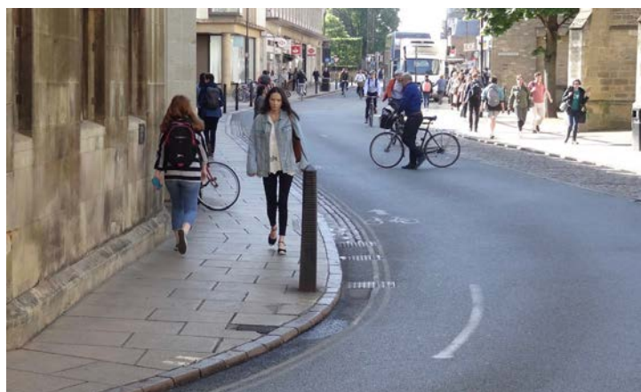
Image 66: Poorly Maintained Cycle Lane ending at Junction in St. Andrew's Street
