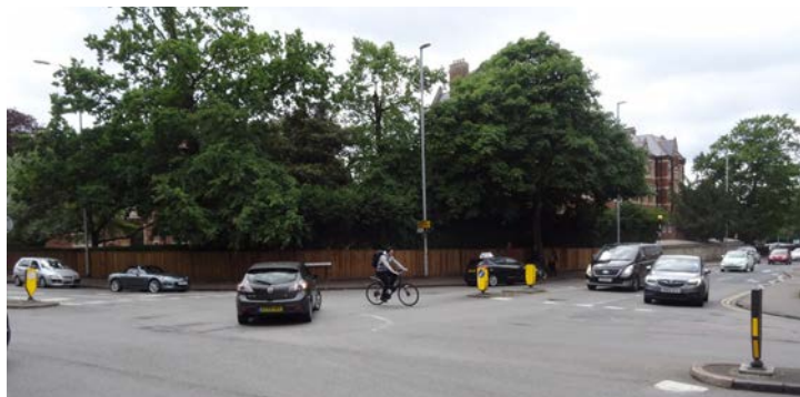
Image 67: Safety Concerns at Trumpington Street Mini-Roundabout
