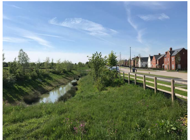
Sustainable Drainage Systems
