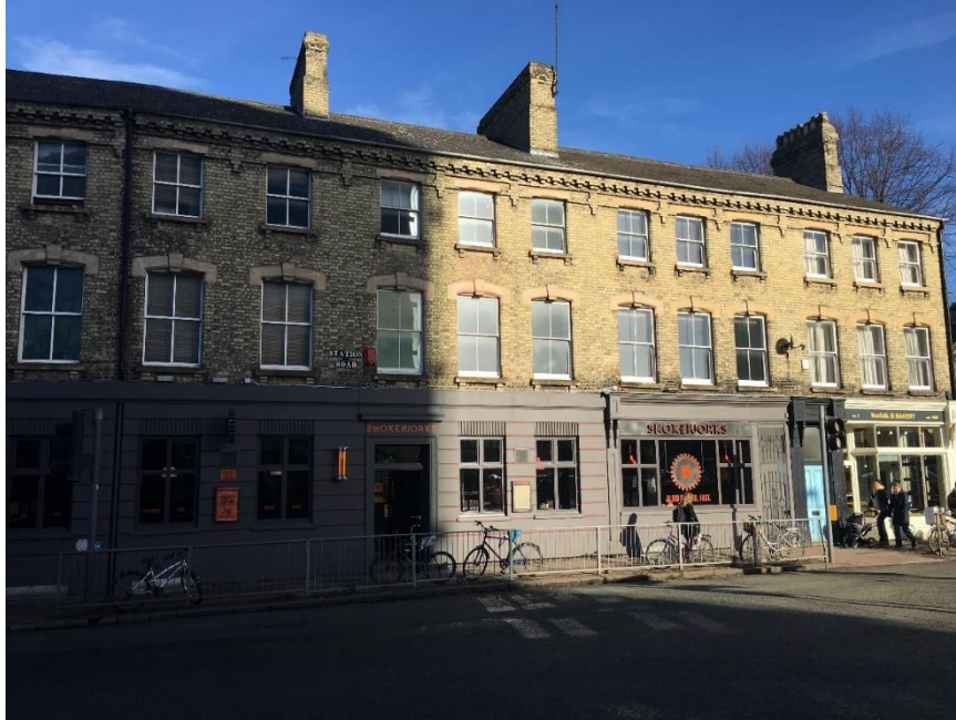
Figure 18: view of 5 - 7 Hills Road
