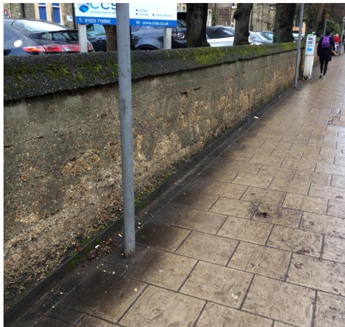
Figure 17: No-fines Concrete Wall
