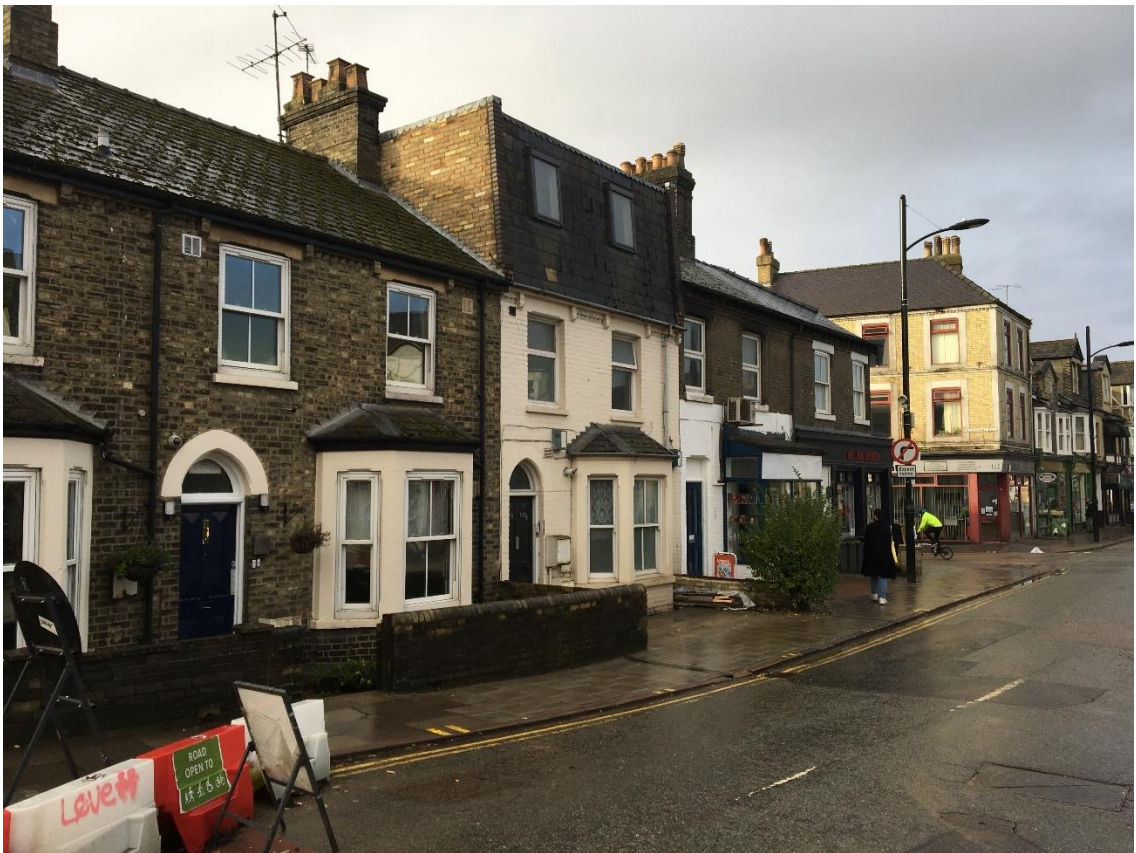
Figure 16 View of nos. 120-112 Mill Road
