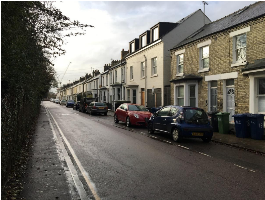
Figure 17 View of the Devonshire Road Terrace with the site boundary seen on the left of the photograph
