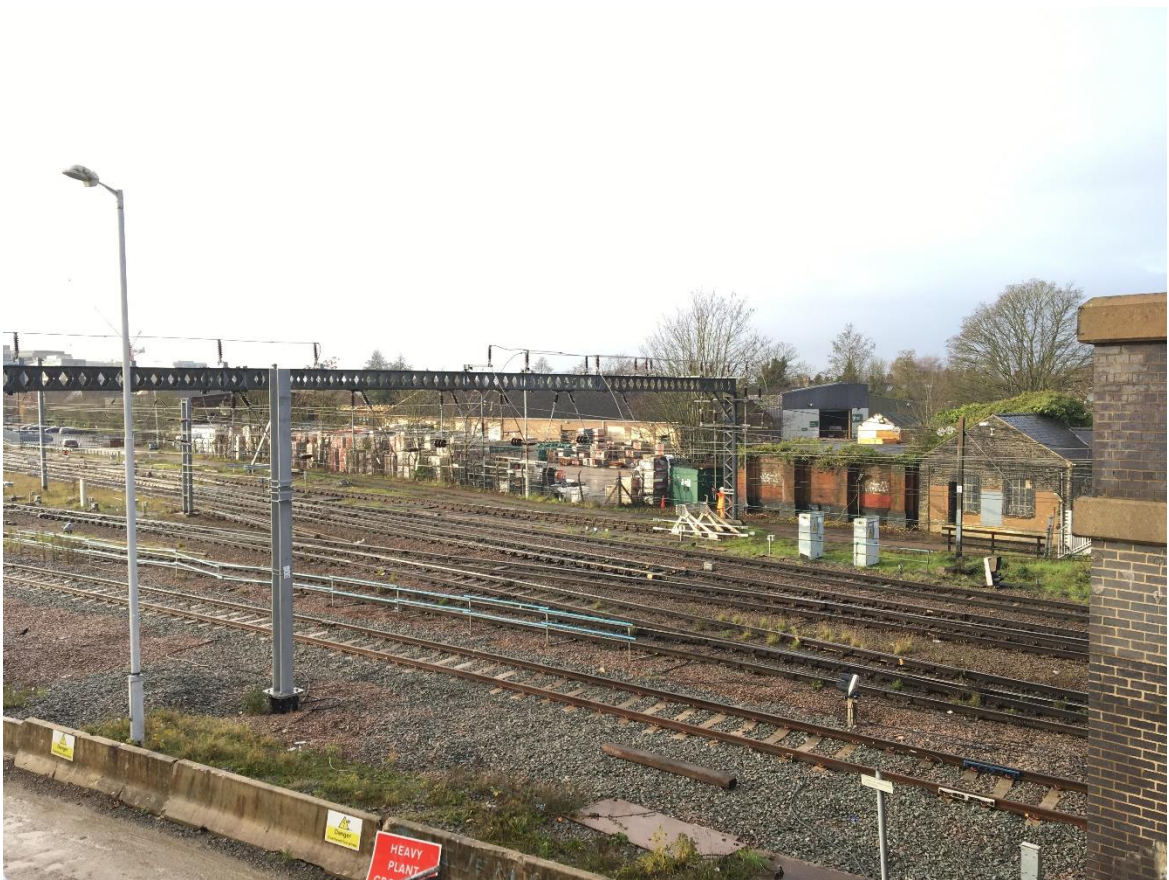
Figure 11 View of the site as seen from the east of the railway bridge
