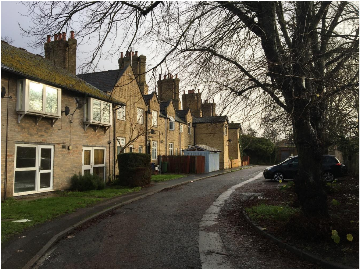
Figure 13 View of the southern elevation of nos. 126-134 Mill Road
