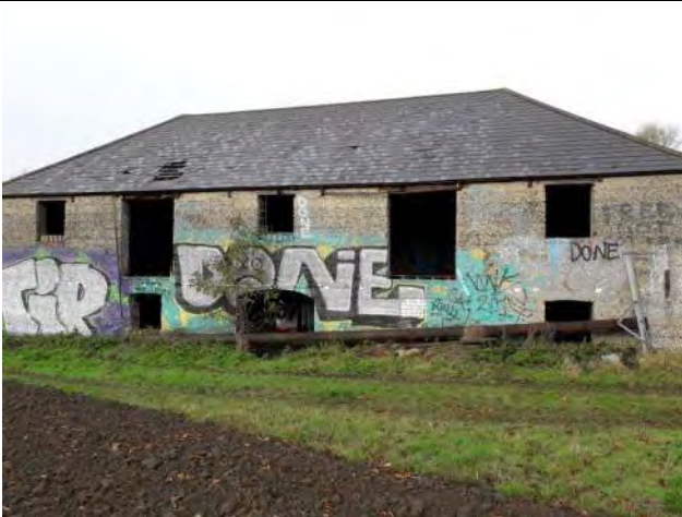
Photo 5: Building 1, Foxton South, high bat potential, external view.
