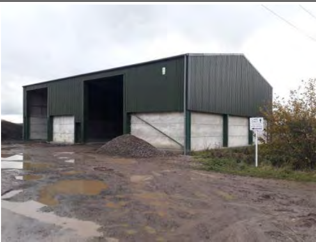
Photo 3: Building 2, Foxton North, Medium bat potential.
