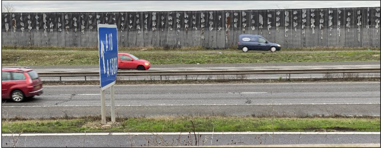
Figure 4—6 Existing M11 barrier
