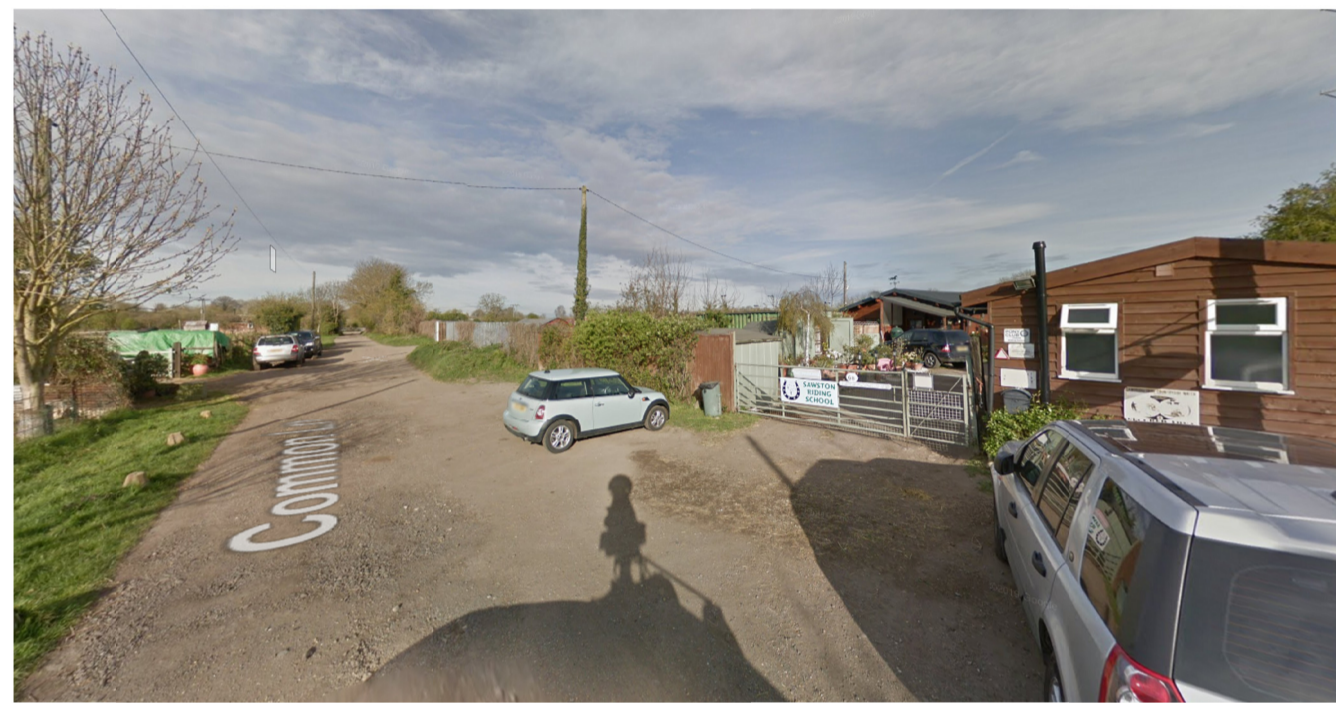
View of Riding School on Site from Common Lane
