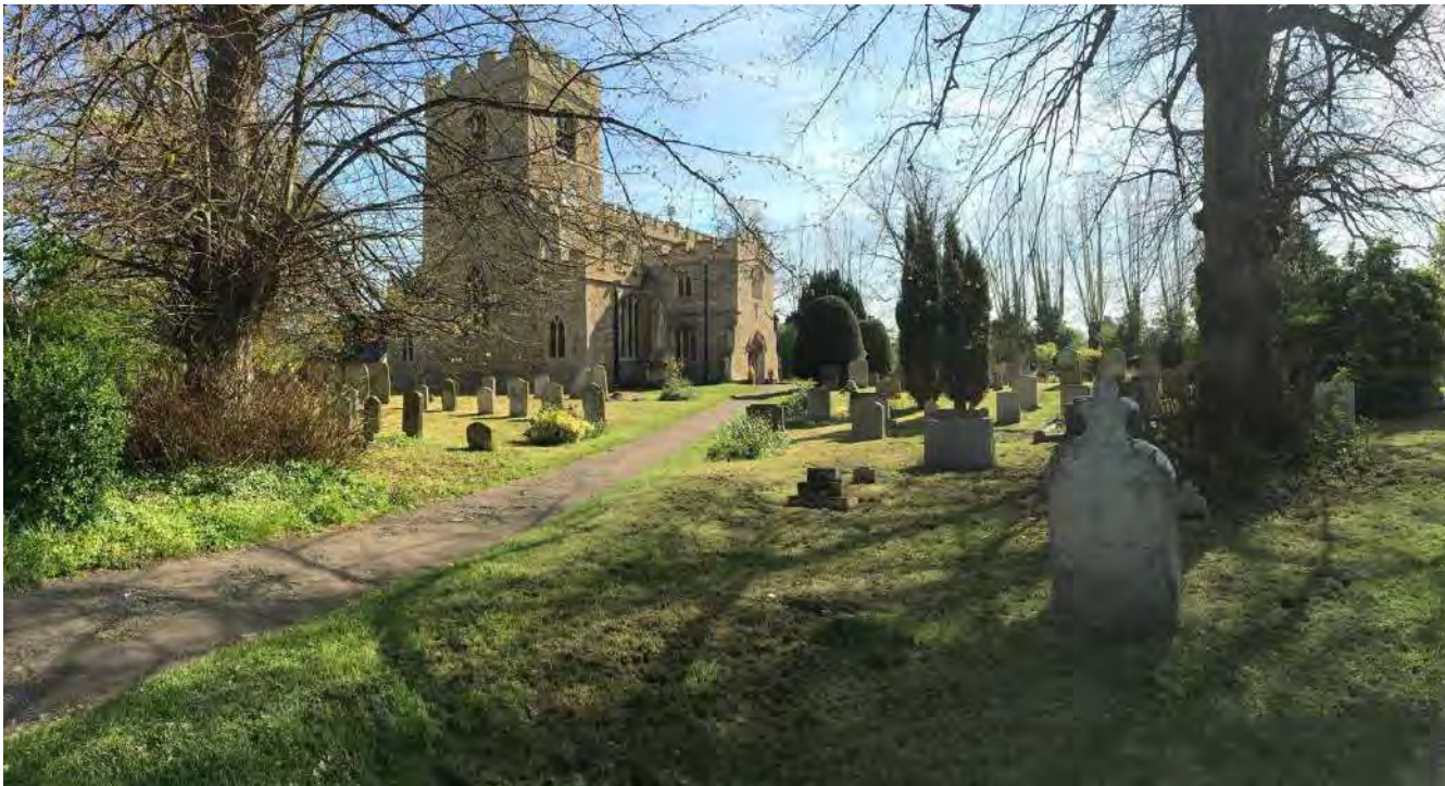
The Parish Church of St Andrew, Girton
