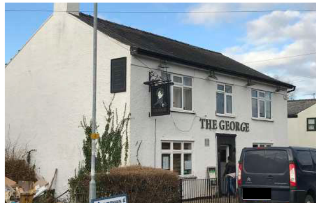
The George Pub & Thai Restaurant is located on High Street to the west of the Site, within a 5 minute walk.
