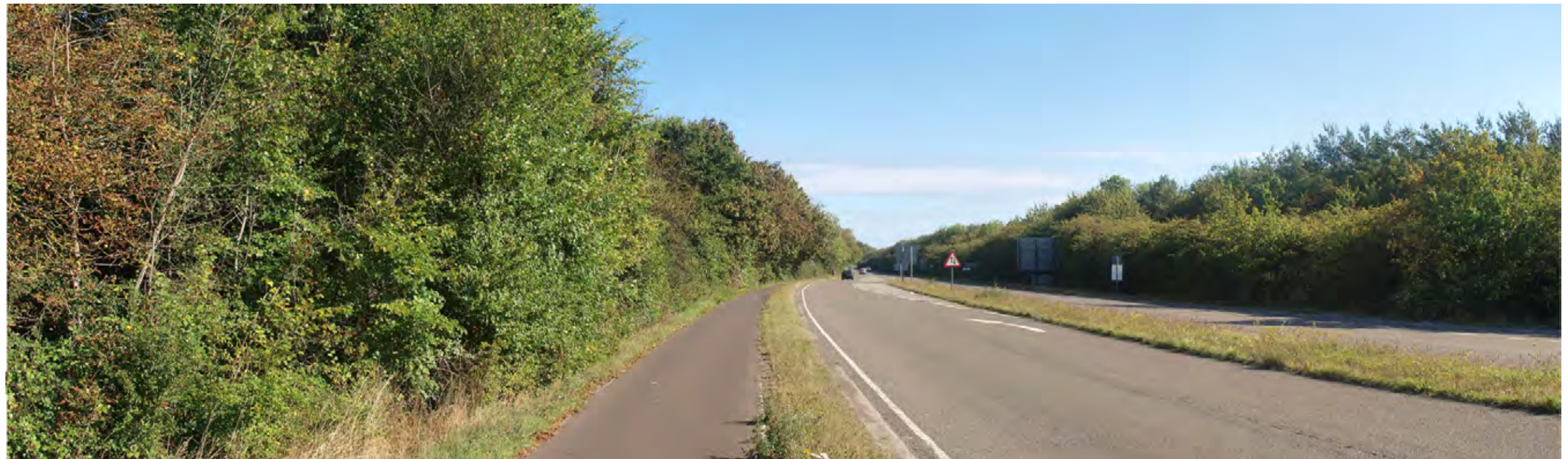
View from Barton Road looking north-east - Viewpoint B
