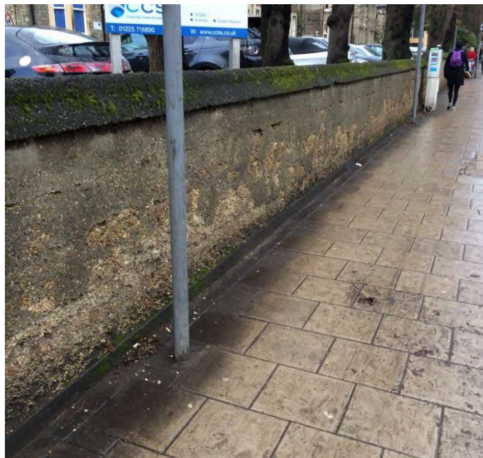
Figure 17: No-fines Concrete Wall
