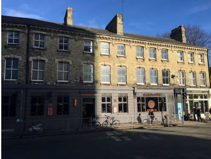
Figure 18: view of 5 - 7 Hills Road
