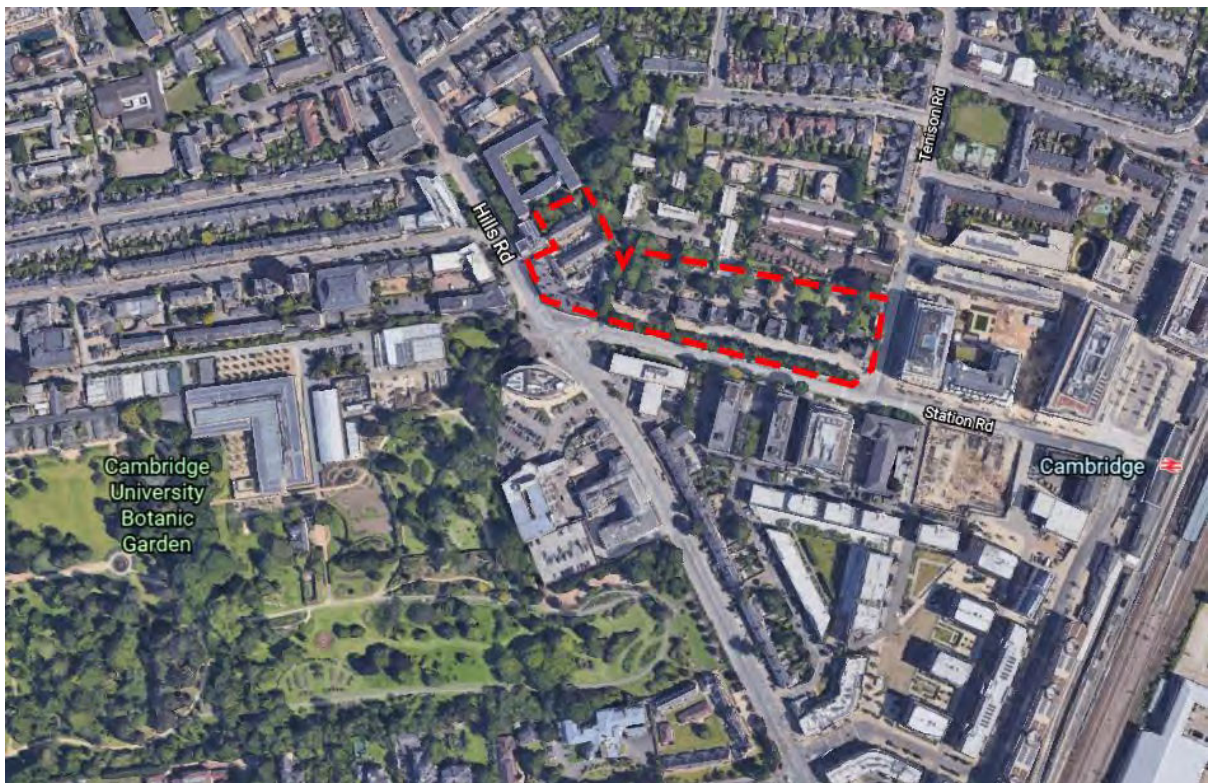
Figure 1 Aerial demonstrating the location of the site. the approximate boundary of the site is marked in red
