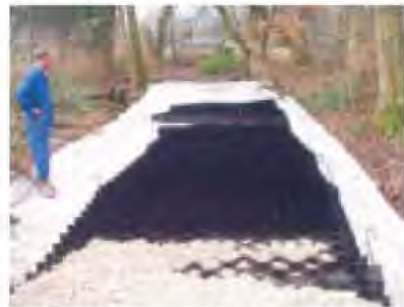
Installation of the CellWeb™ system.
