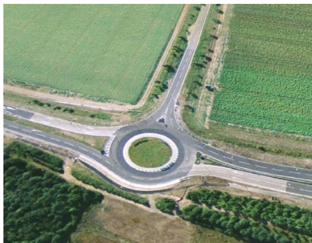
A505 Hunts Road junction (Google Earth)
