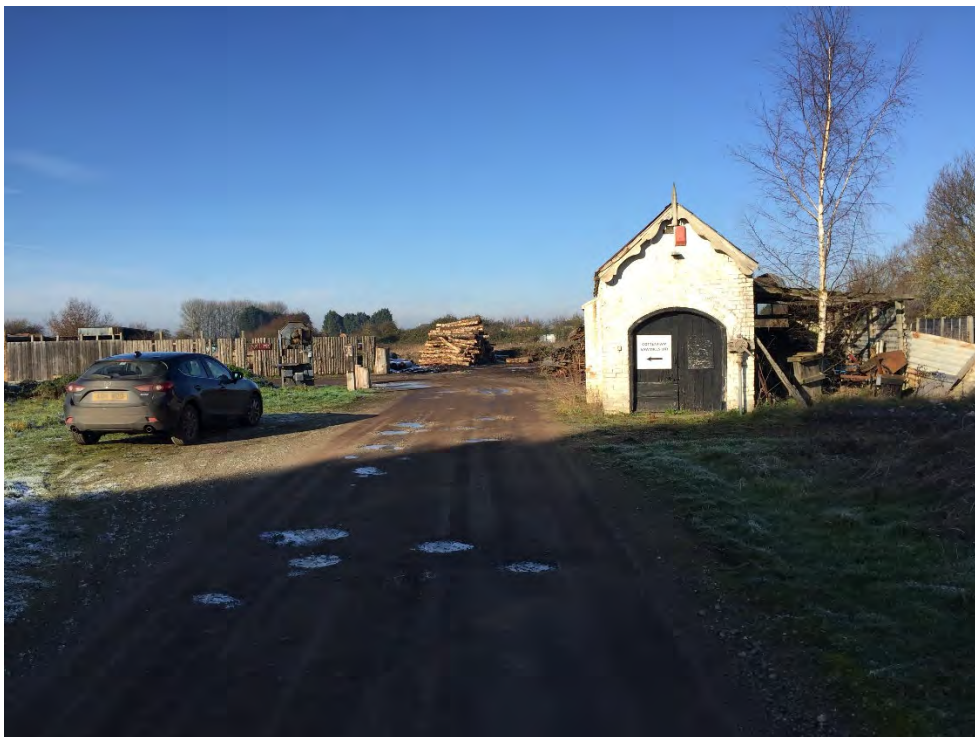
Fig 4 – parking, storage, fencing and brick building
