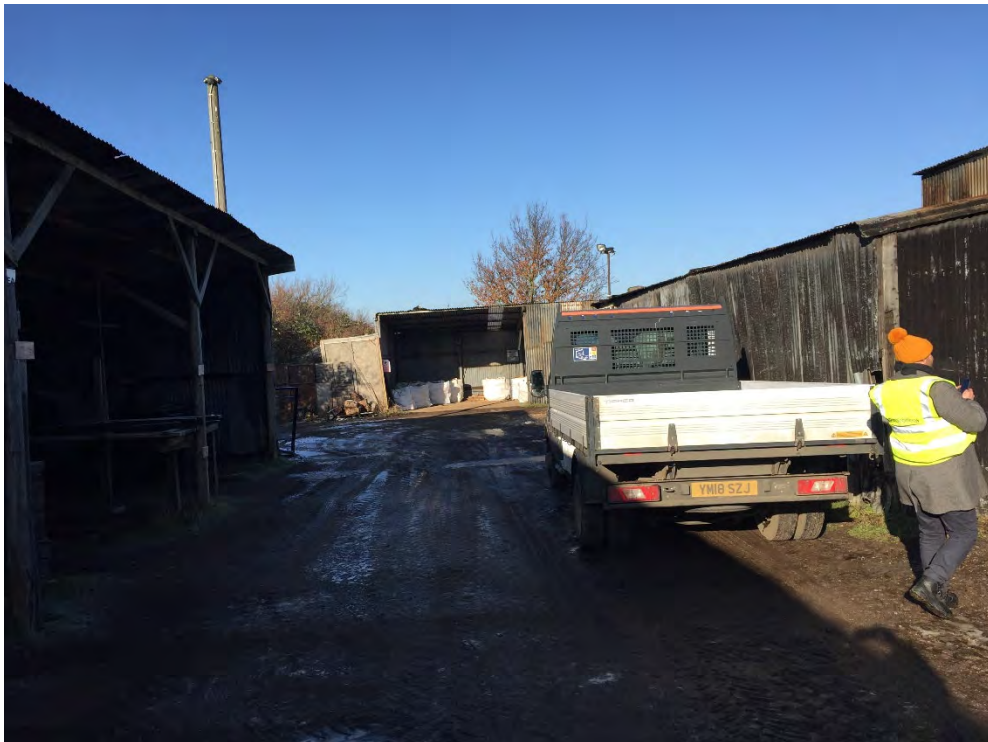
Fig 8 – Internal site road
