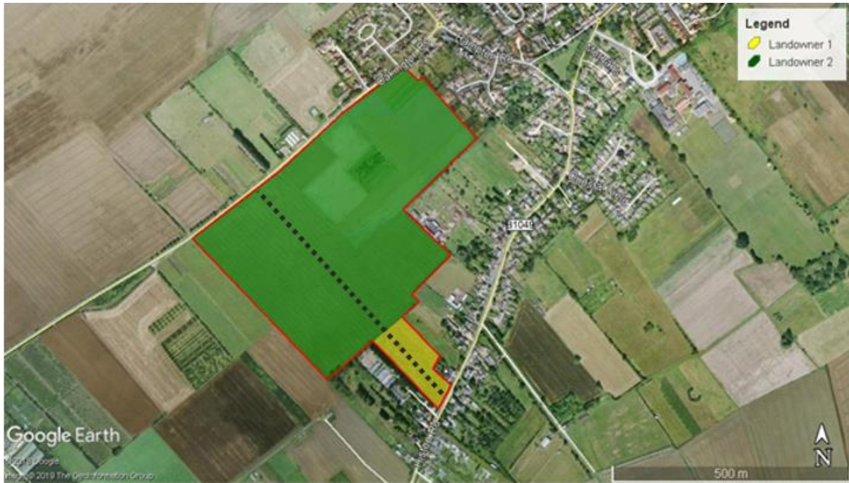
Figure 3: Showing access to the site via Histon road and Oakington road.
