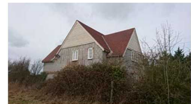
New dwelling under construction to the North of the site.
