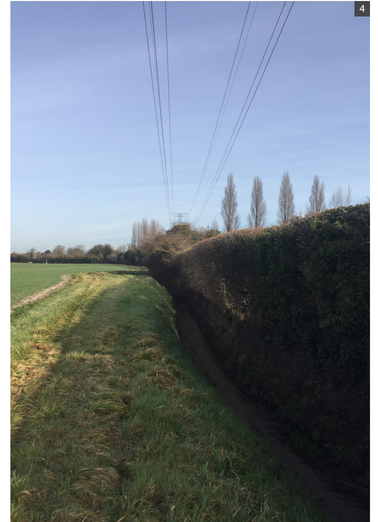
High voltage power cables follow the alignment of hedges and ditches
