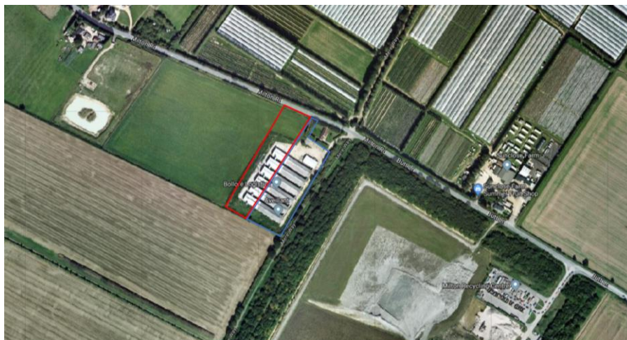
Figure 1: Site Location Plan showing the former poultry sheds before their conversion
