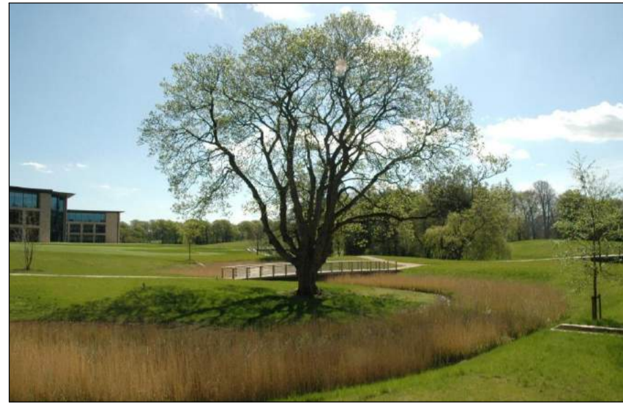
INFILTRATION/ATTENUATION BASIN: BASINS WILL PROVIDE ATTENUATION AND TREATMENT OF STORMWATER AS WELL AS AMENITY AND BIODIVERSITY SPACE.
