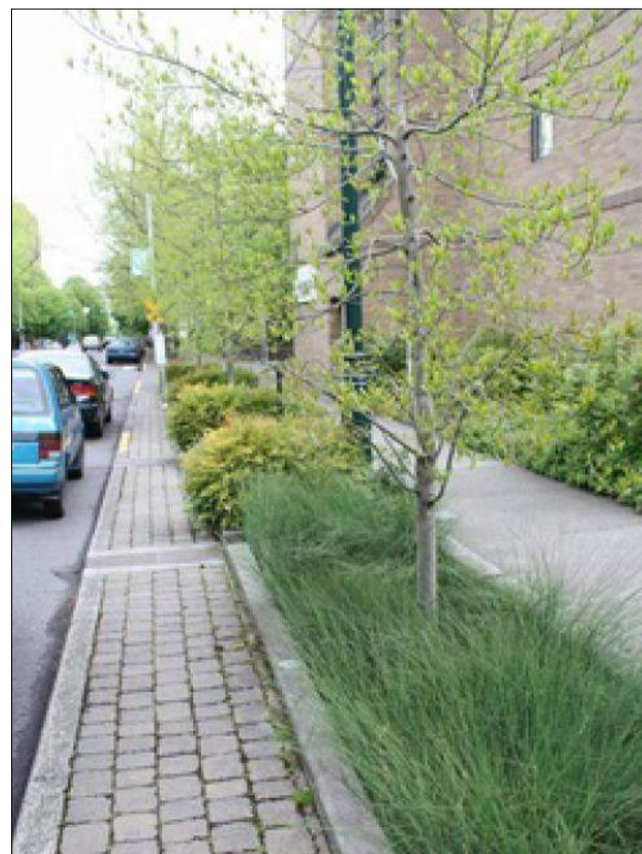
BIO RETENTION AREAS: BIO RETENTION PROVIDES A SMALL AMOUNT OF UPSTREAM STORAGE AS WELL AS AN ADDITIONAL SURFACE WATER TREATMENT STAGE PRIOR TO DISCHARGE.
