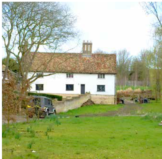
Grade II Listed Old Victorian Farmhouse
