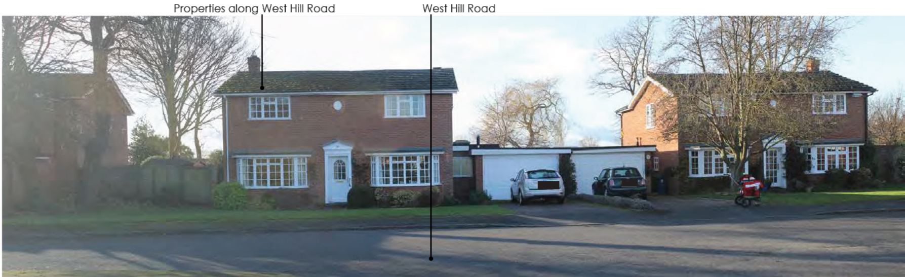
View from West Hill Road looking south-west towards the Site Photograph 08
