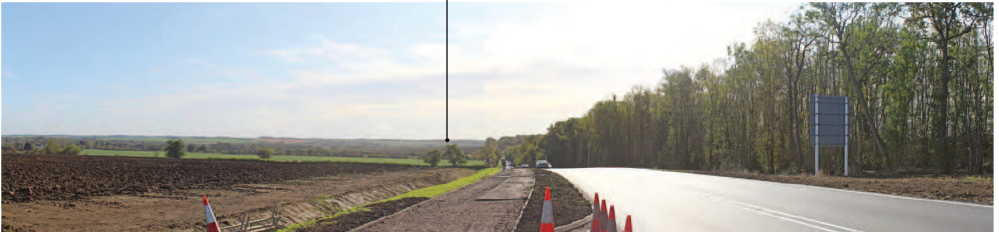
View from the A1198 looking south east towards the Site Photograph 25
