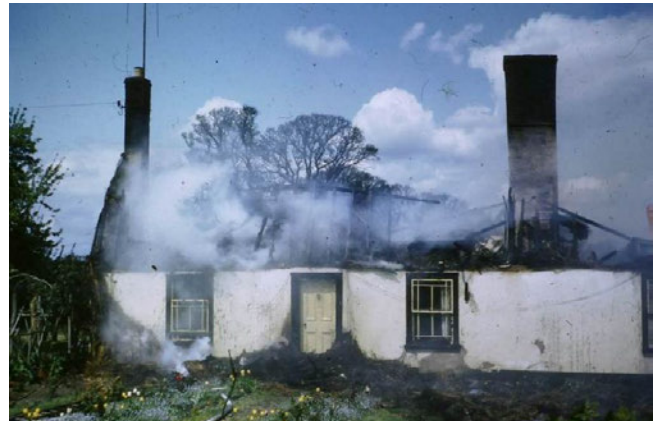
Destroyed by fire ca. 1960 4
