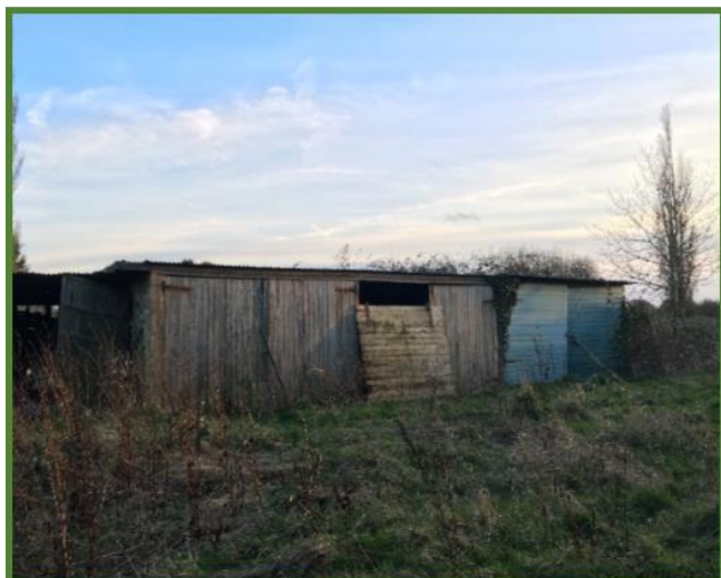
Figure 7: Disused agricultural building
