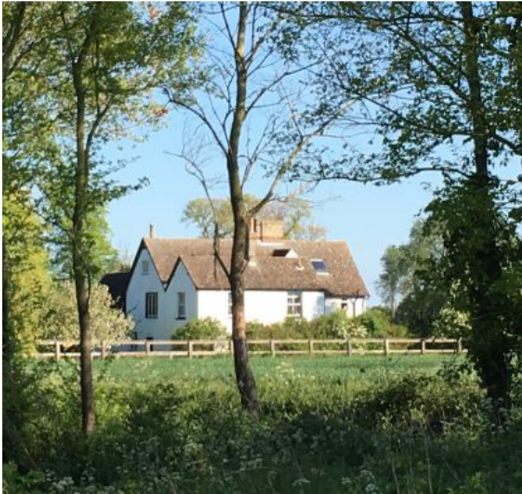
Figure 8 - St John's Farmhouse, seen from the rear.
