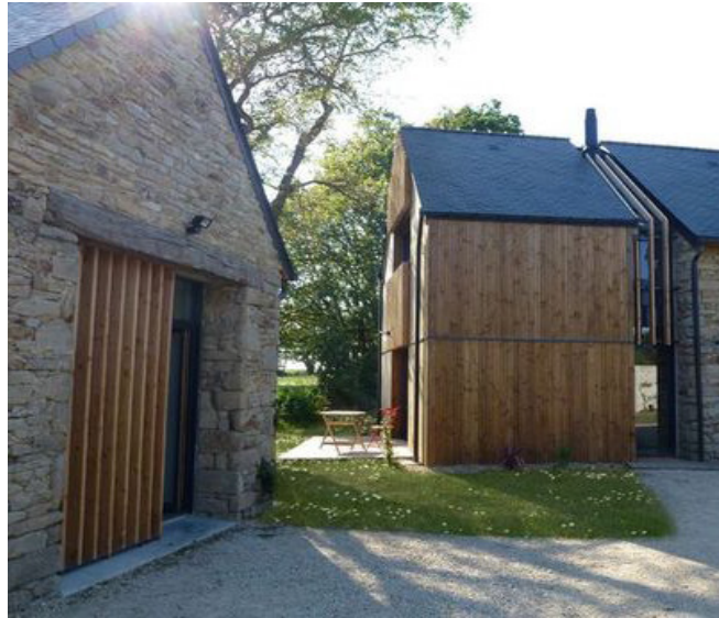
Figure 38; Example of relationship between buildings and longer views between
