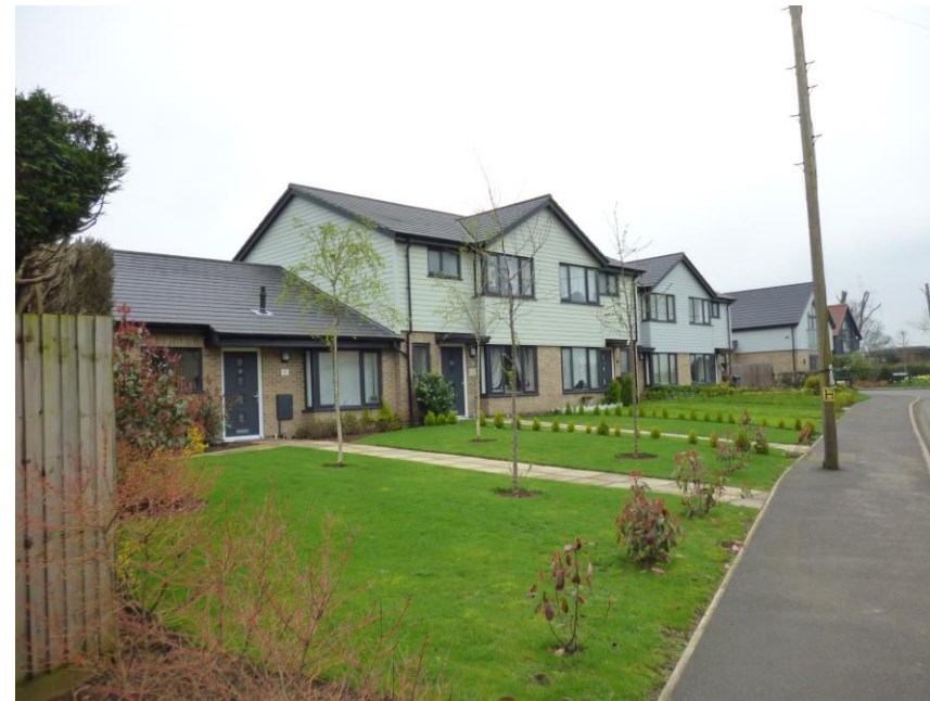
New residential development along Cinques Road
