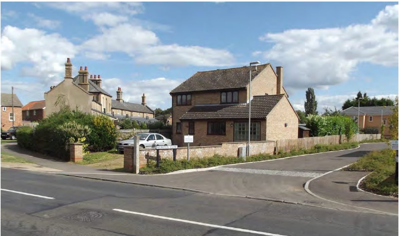
Plate 6: View from Oakington Road, showing relationship of new development at Moreton Close and Listed almshouses (Sept 2012)
