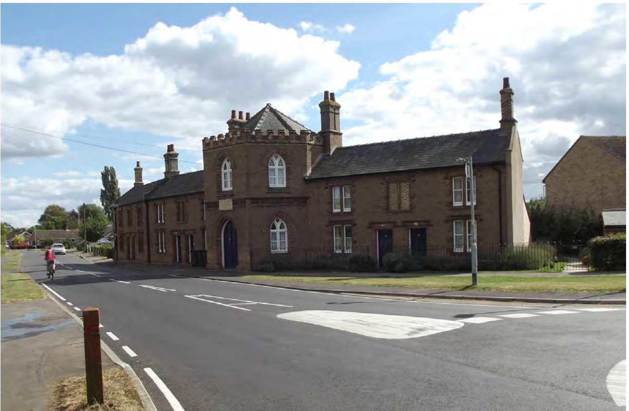
Plate 4: Moreton's Charity Almshouses (looking southeast from Rampton Road) (Sept 2012)
