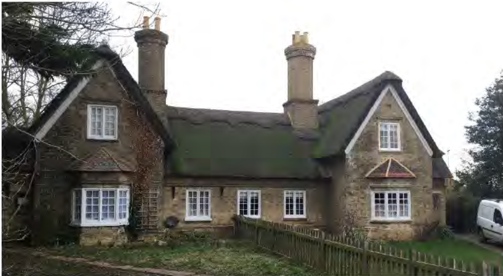
Figure 13 - 20 and 22 Church Lane.
