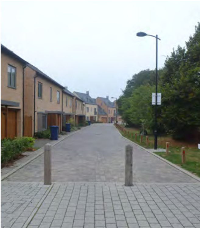
Figure 46; Housing facing woodlands
