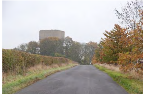
The water tower to the west of Cockayne Hatley is a prominent landmark
