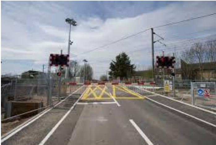
Figure 4 – Fen Road Level Crossing
