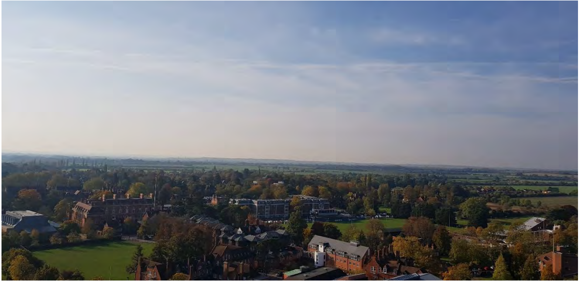
Figure 19 View looking south-west
