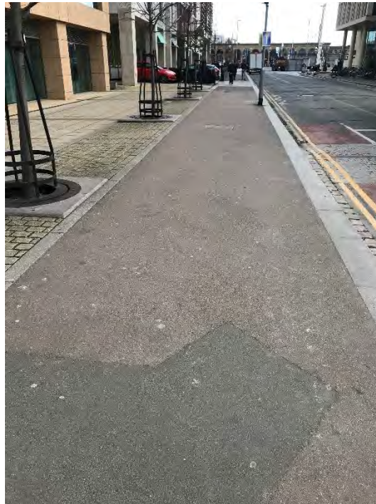
Figure 10: Footways Along Station Road, Outside CB1 Development
