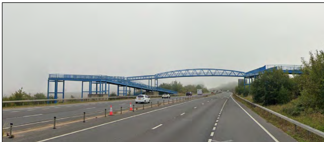
Photo 4.1 Existing Foot-Cycle Bridge
