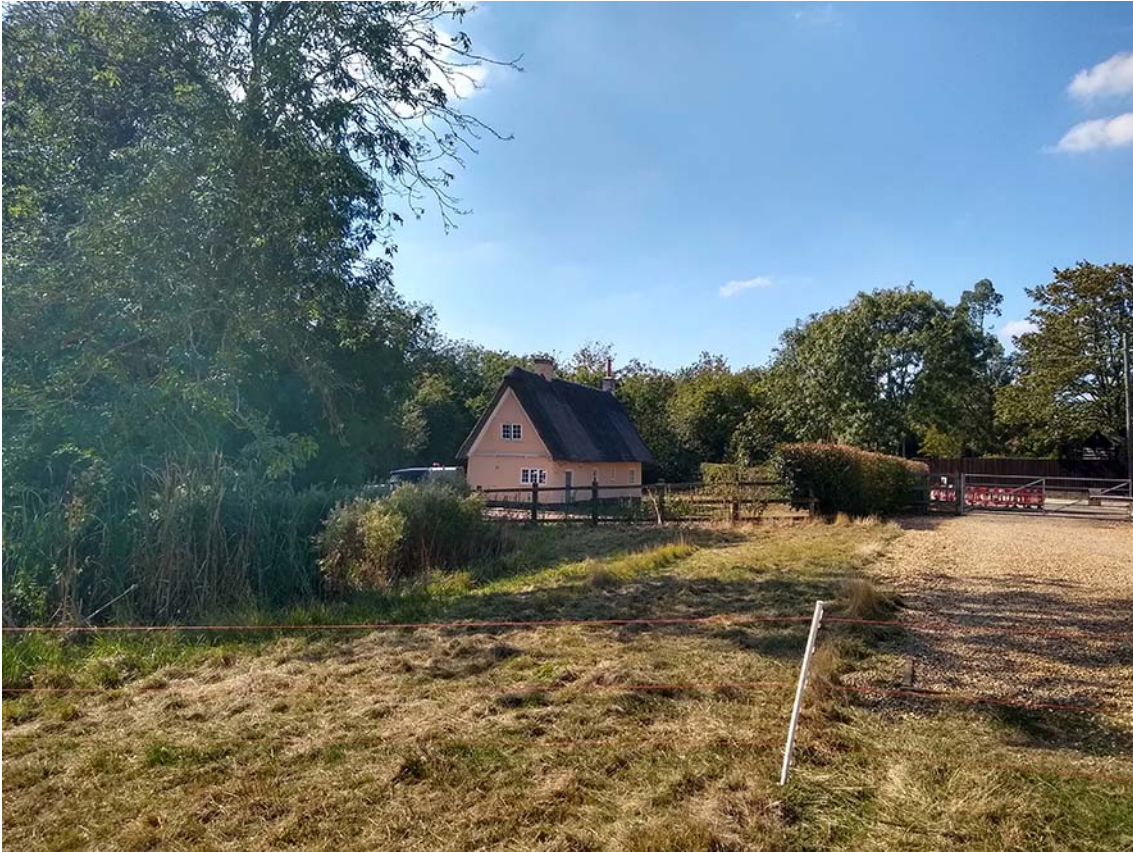
Plate 7. Victoria Farm Cottage (Grade II listed) in south-western corner of northern area
