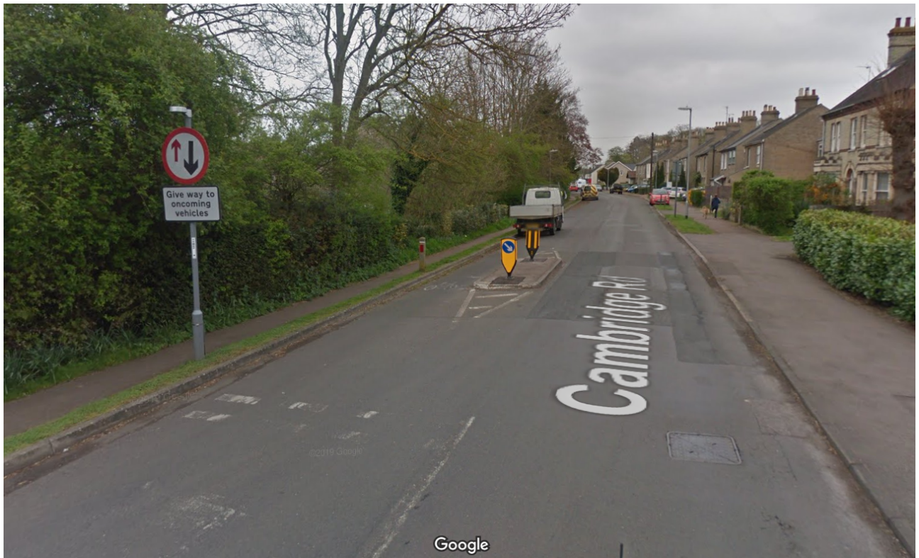
Figure 9: Cycling Route / Traffic Calming on Cambridge Road (Looking North)
