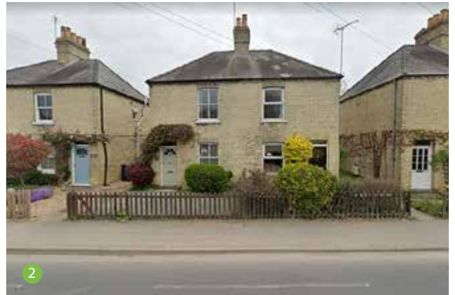
Bridge Road |(North)
