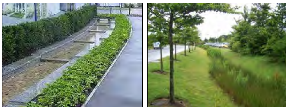
Figure 7.4: Open Swale / Rills Example
