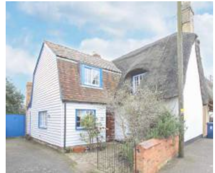
Figure 25: Thatched roof house with white cladding
