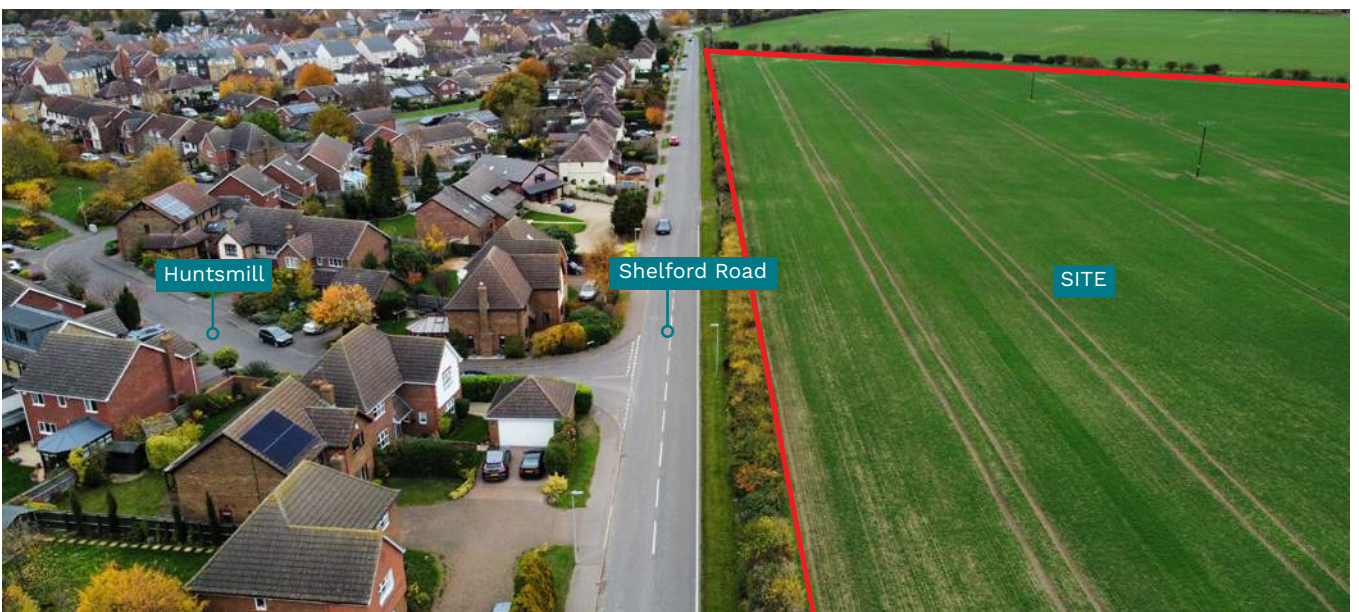
View looking north-east along Shelford Road
