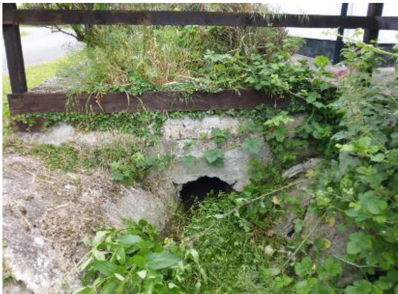
Top: Inlet Looking Downstream Bottom: Outlet Looking Upstream
