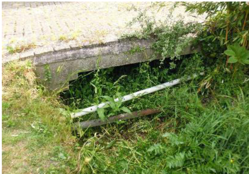
Top: Inlet Looking Downstream Bottom: Outlet Looking Upstream
