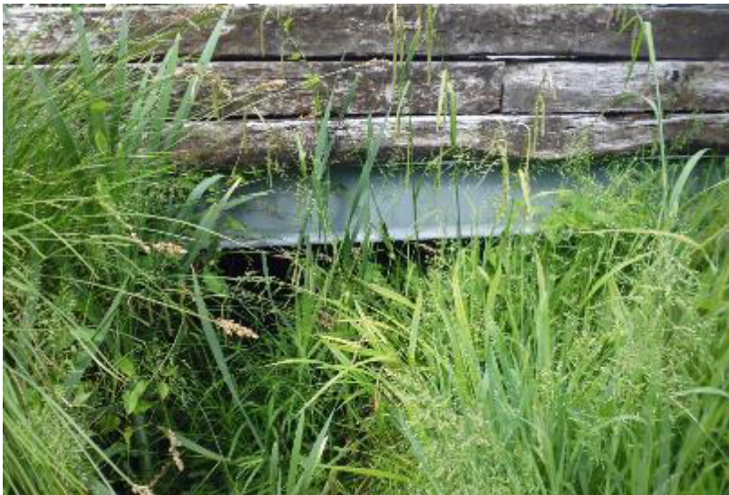
Top: Inlet Looking Downstream Bottom: Outlet Looking Upstream
