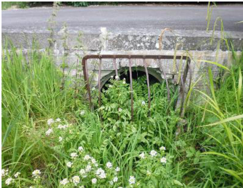
Top: Outlet Looking Upstream Bottom: Inlet Looking Downstream
