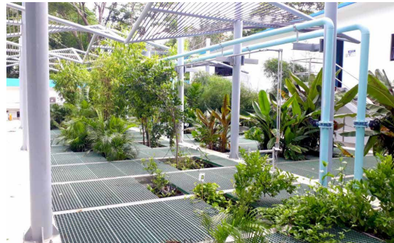
Example of food chain reactor for onsite wastewater treatment and recycling, that is odourless and contributes an indoor garden to light industrial Technopark (source Organica)
