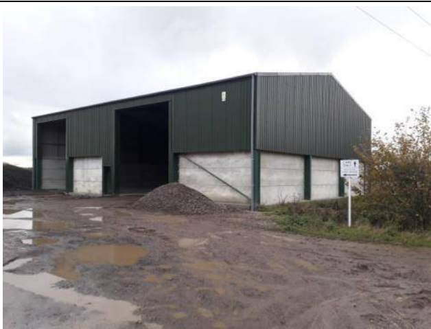
Photo 3: Building 2, Foxton North, Medium bat potential.
