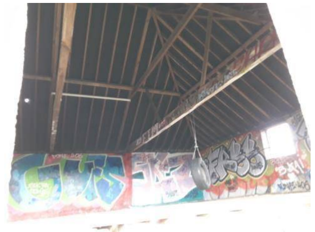
Photo 6: Building 1, Foxton South, high bat potential, internal view.
