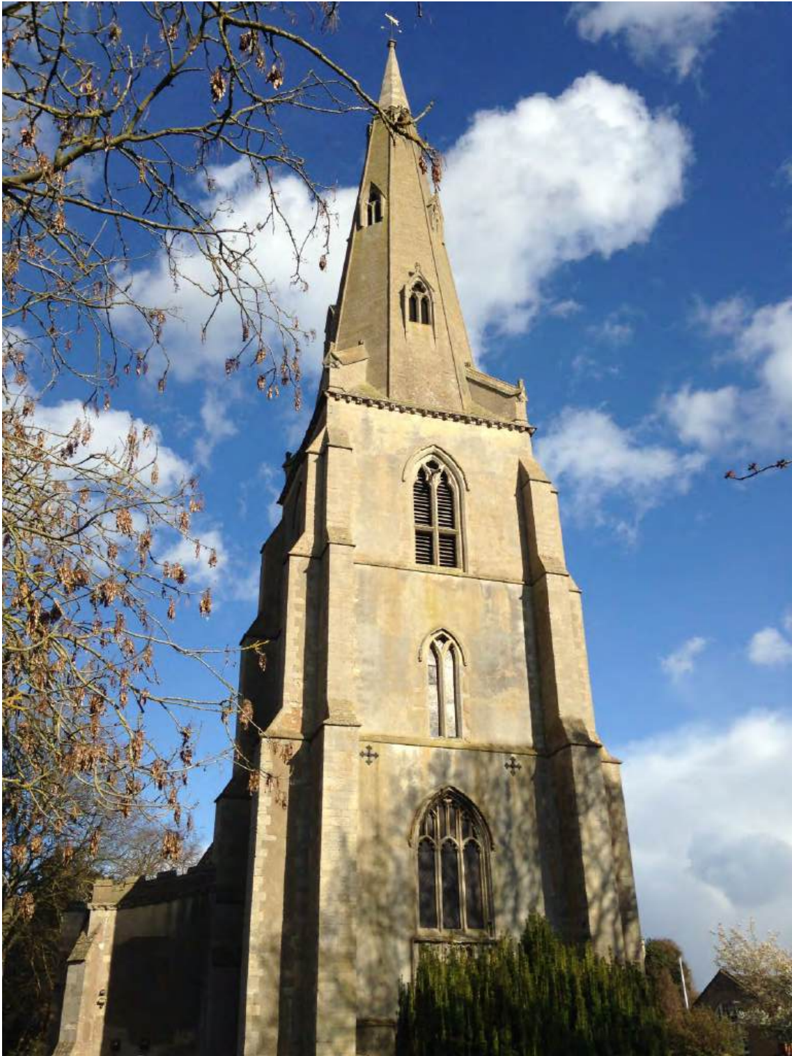
Plate 9: Church of St Marys (tower and spire), Over (Grade I Listed Building, NHLE entry: 1317811) from the western end of the churchyard.
